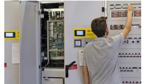
FAT, Start-up & Commissioning
